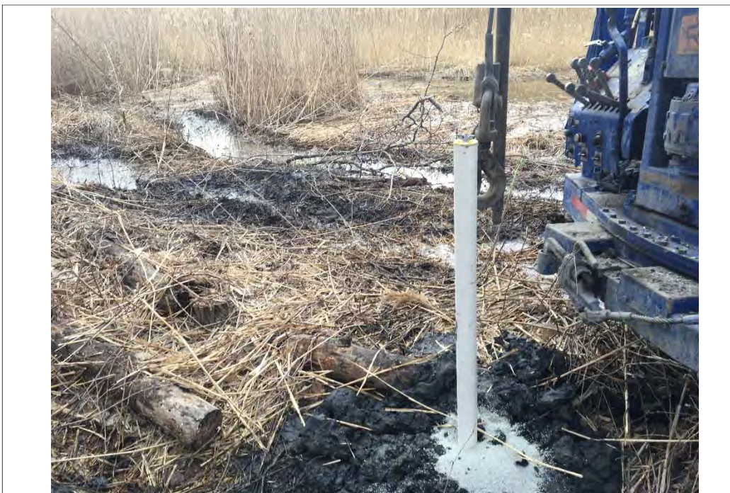
Temporary Monitoring Well MW-3.
