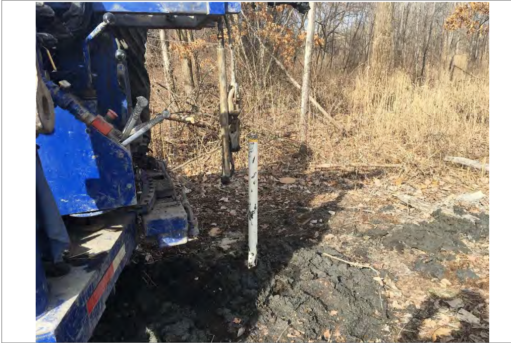
Temporary Monitoring Well MW-2.
