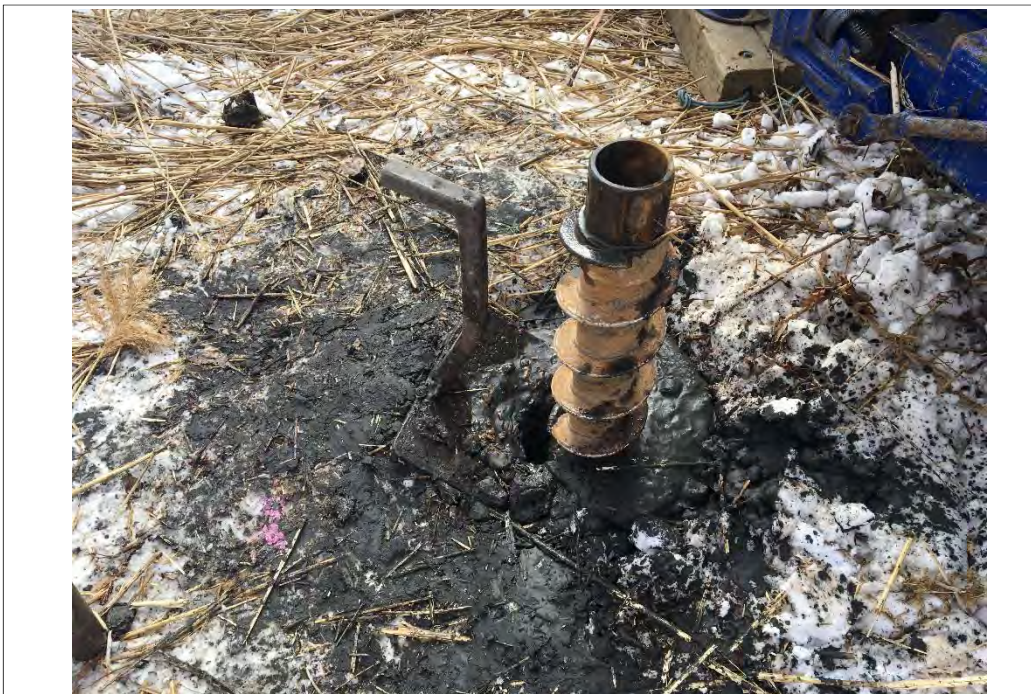
Hollow Stem Auger at B-4 Location.
