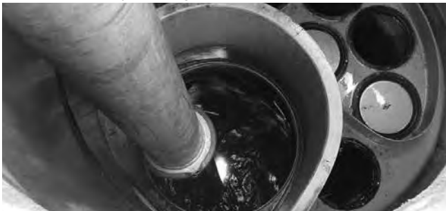
Vacuuming Sump Through MAW
