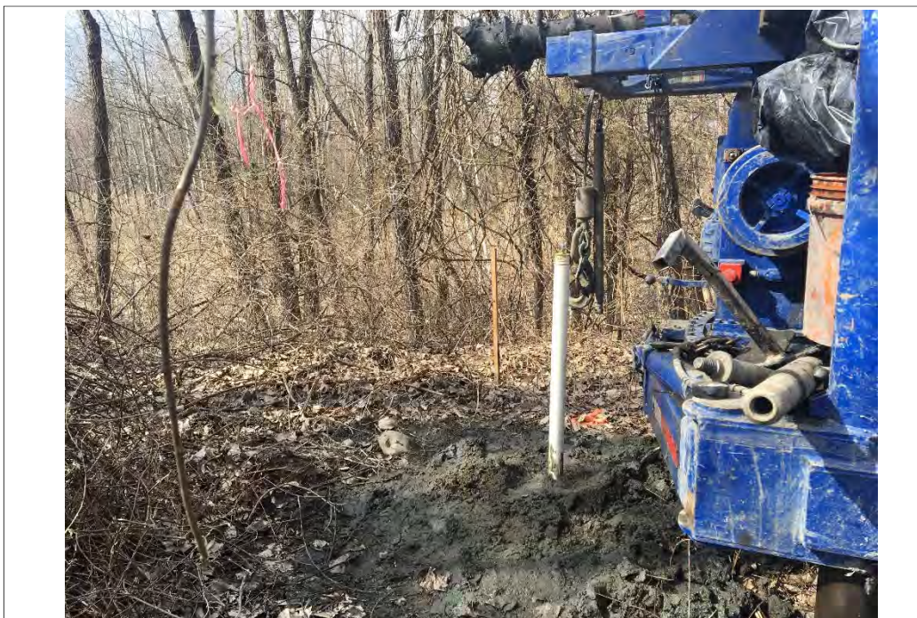
Temporary Monitoring Well MW-1.
