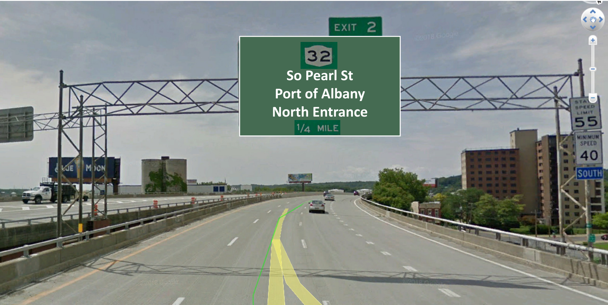
Reference Location 1: Interstate 787 South Bound Approaching Exit 2
