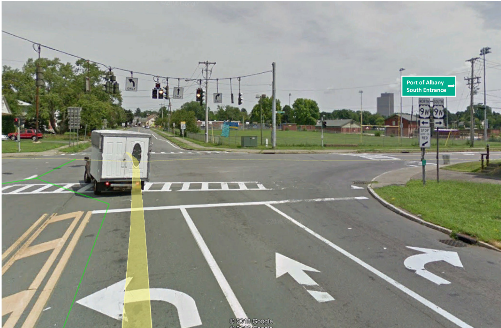
Reference Location 14: Interstate 787 South Exit 1 at Route 9w
